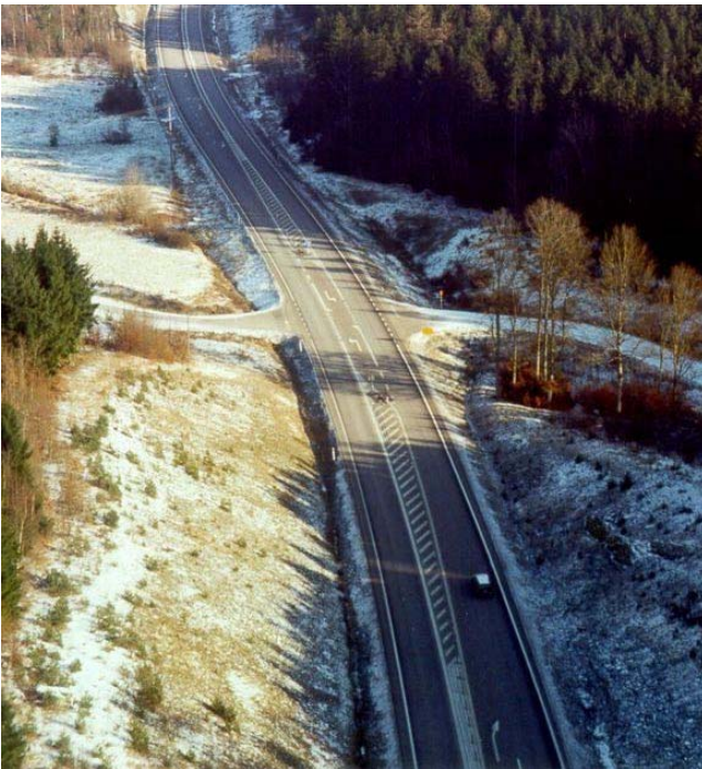
Figure 24. Four-legged intersection on 2+1 roadway in Sweden.
