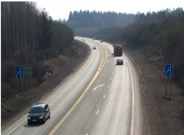
Figure 14. Example of a lane-drop transition in Finland.
