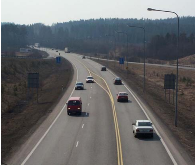
Figure 13. Example of a lane-addition transition in Finland.
