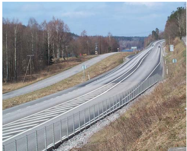
Figure 25. Example of a noncritical transition in Sweden.
