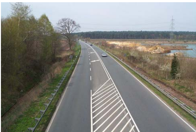
Figure 2. 2+1 roadway in Germany.
