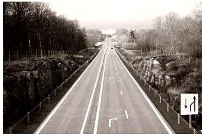
Figure 27. Example of a critical transition in Sweden.
