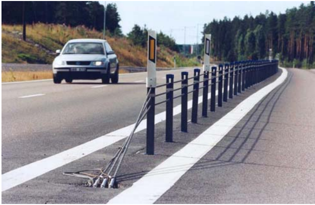
Figure 19. Cable barrier end treatment in Sweden.
